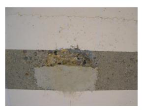
Re-profile using S&P Resin 230 HP levelling mortar.
