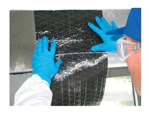
Fix the pre-impregnated S&P C-Sheet 640 onto the substrate.
