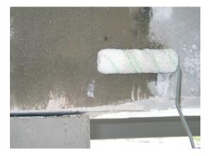
Apply S&P Resin 55 HP (vapour proof) onto the substrate.
