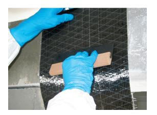
Pull the rubber spatula, always in the direction of the fibres, until all fibres are moistened and there are no air pockets left in the sheet.
