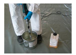
Mix S&P Resin 55 HP at a low speed, max. 400 RPM.
