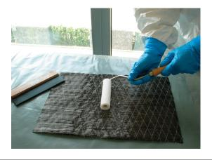
Pre-impregnate the S&P C-Sheet 640 with S&P Resin 55 HP. Laminate the mesh in the direction of the fibred by spreading the resin evenly with a rubber spatula (S&P squeeze) and a Teflon press roller.
