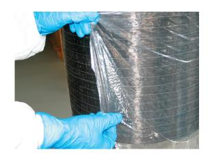
Fix the pre-impregnated S&P C-Sheet 240 onto the substrate, remove protective film and laminate with a rubber spatula (S&P Squeeze) or press roller.
