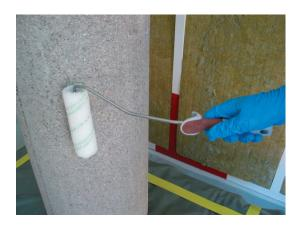
Apply S&P Resicem HP (improves vapour exchanges) or S&P Resin 55 HP (vapour proof) onto the substrate.
