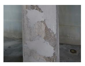
Remove bad concrete (honeycomb), masonry, loose material, wood pieces, insulation material etc.
