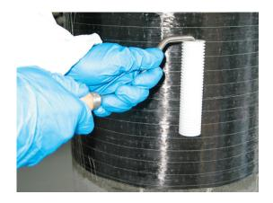
Always roll in the direction of the fibre, ad do so until all fibres are moistened and there are no air pockets left in the sheet.
