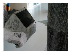
In this stage of work, also cover the sheets' area in quartz sand. This will act as a rough course to ensure the adhesion of plaster or mortar later on.
