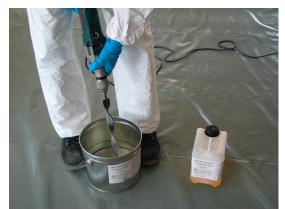
Mix the adhesive at a low speed, max. 400 RPM.
