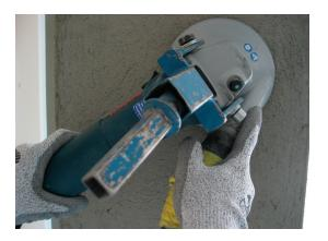
Sand blast, shut blast, or grind the substrate using a cup wheel. Not using a chisel!
