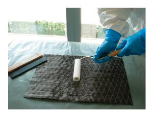
Pre-impregnate the S&P C-Sheet 240 with S&P Resicem HP or S&P Resin 55 HP.
