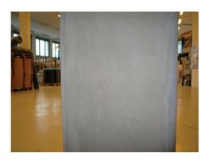
Re-profile using S&P Tecnogrout-K or S&P Resin 230 HP.
