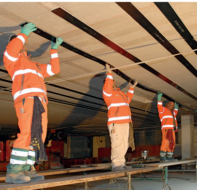
Surface applied S&P C-Laminate (Bending)
