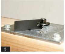
5. Check to ensure the proper engagement of the TUW tabs to the SDWF screw shank using the screw depth guide (provided). The measured gap shall be no greater than 7mm and no less than 4mm.
