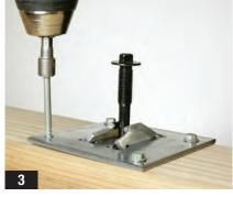
3. Secure the TUW to the upper-wall bottom plate with (4) SD#9 x 64mm Simpson Strong-Tie® Strong-Drive® SD Connector screws (provided).
