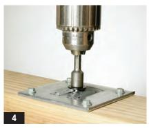
4. Continue driving the SDWF screw until the washer head contacts the threaded TUW tabs and bends them until they engage the shank of the SDWF directly under the head. Do not overdrive!
