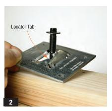
Slide the TUW (provided) over the SDWF screw head and center using locator tab as a reference. Orient locator tab so that it points toward the outside of the wall.
