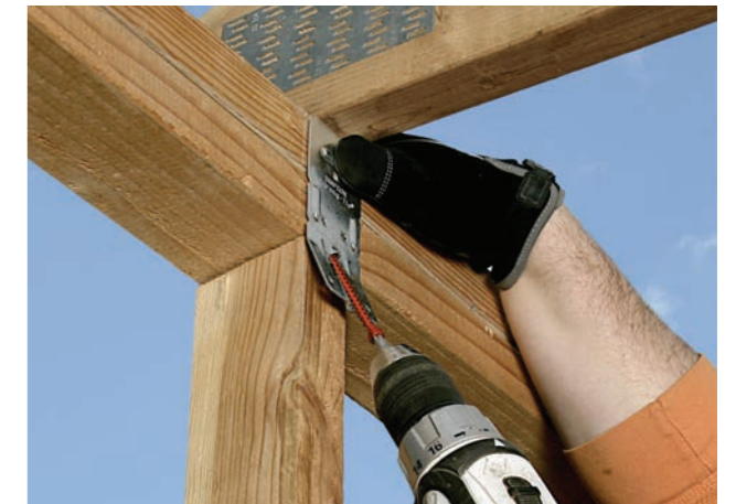
STEP 2 – While continuing to drive the SDWC, “drop” the fastener head into the guide channel to ensure optimal installation angle of 22°. The installation angle range is 10°–30° (see illustration). Once the installation angle is established, the metal installation guide tool may be removed.
