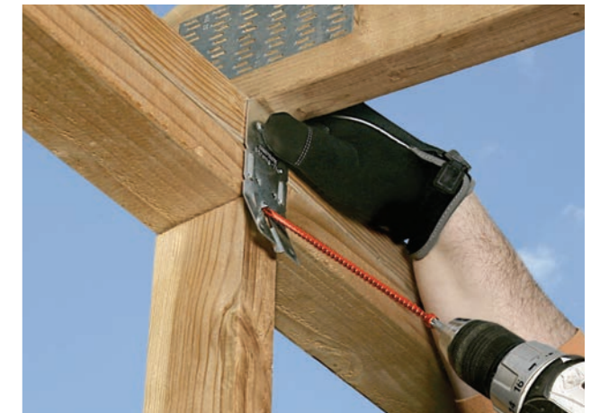
STEP 1 – Align the metal installation guide tool (included) with the truss, and drive the tip of the Strong-Drive SDWC to engage the threads.
