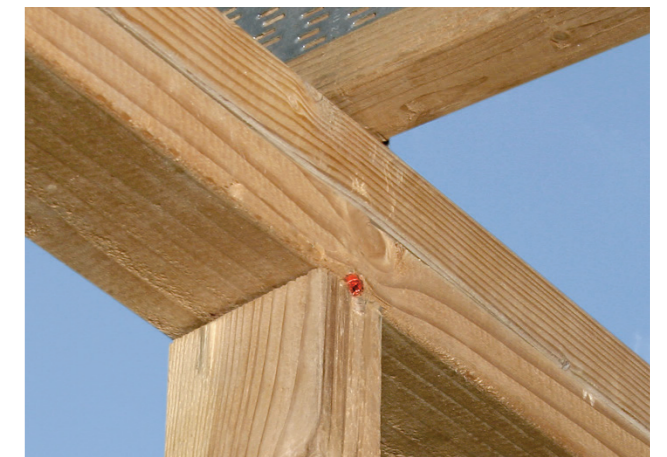
STEP 3 – Drive the SDWC until the head of the fastener is fully countersunk into the double top plate. Verify that the entire shank of the fastener is installed into a timber member.
