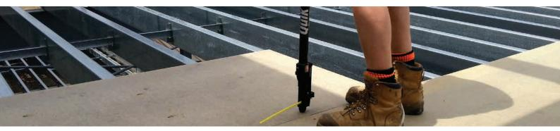
The new Strong-Drive<sup>®</sup> PPSD Subfloor screw has been specifically developed for fastening subfloor sheeting to steel using the Quik Drive<sup>®</sup> auto-feed screw driving system.
