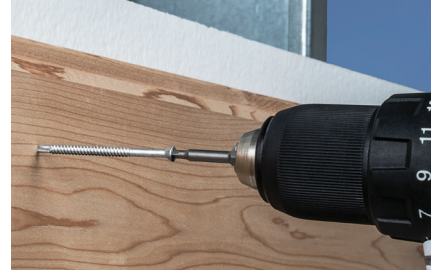
Timber cladding (siding) to steel
