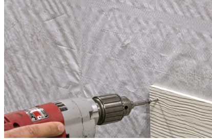
Cement cladding (siding) to steel
