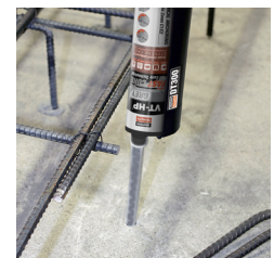
Rebar Doweling
