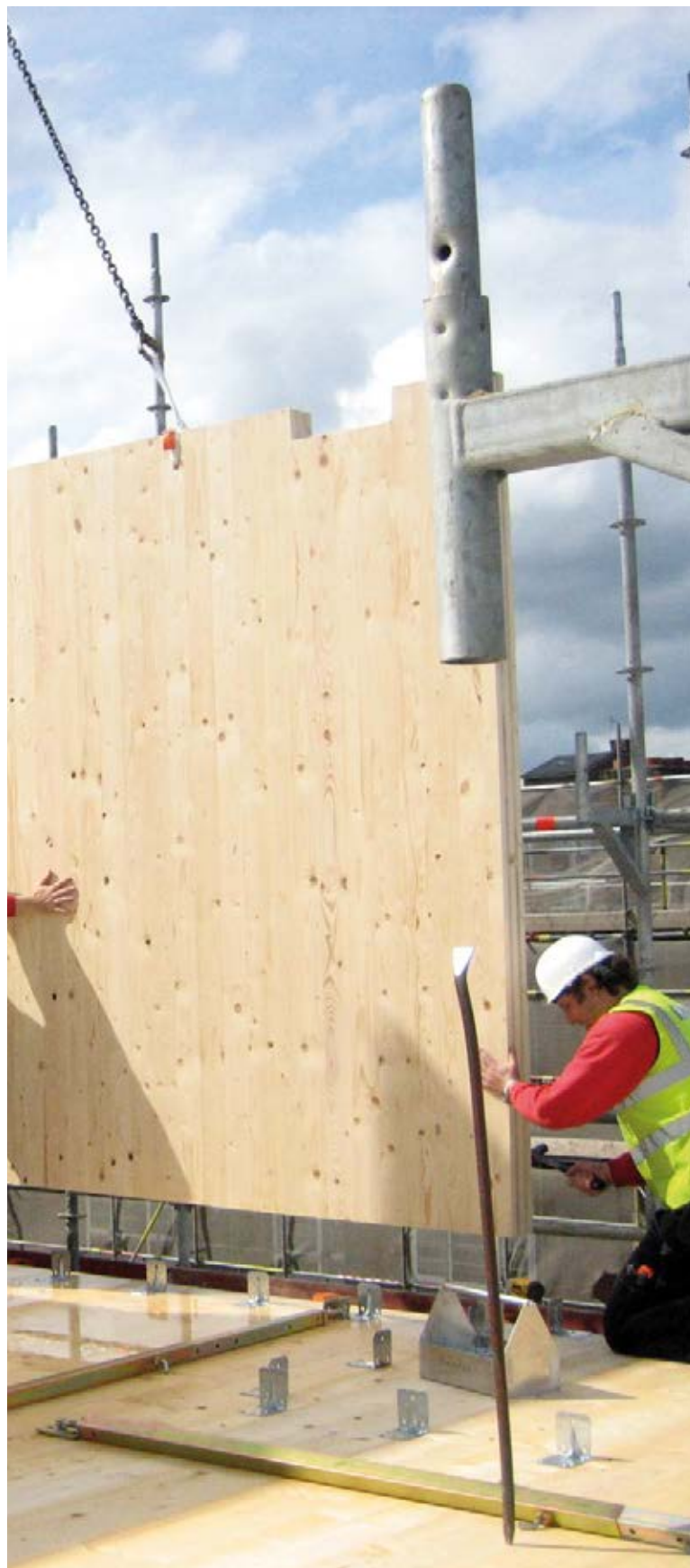
Stadthaus, Murray Grove. Image courtesy of KLH UK.
