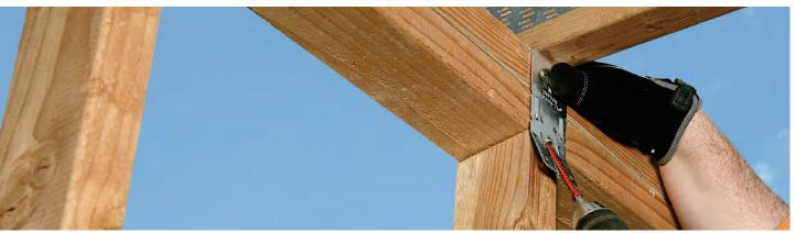
Truss/Rafter-to-Plate and Stud-to-Plate Connection Screws The SDWC Truss screw is tested in accordance with ICC-ES AC233 (screw) and AC13 (wall assembly and roof-to-wall assembly) for uplift and lateral loads between wall plates and vertical wall framing and between the top plate and the roof rafters or trusses. SDWC15450 is recognised for use in chemically treated timber as described in the evaluation report.
