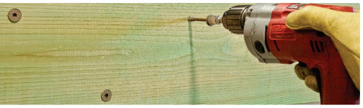
The Strong-Drive® SDWS Timber screw is designed to provide an easy-to-install, high-strength alternative to through-bolting and traditional coach screws. The new SDWS Timber screw is specifically designed for structural timber-to-timber applications and is also ideal for a wide variety of projects where a high-strength attachment is needed – for the contractor and do-it-yourselfer alike.
