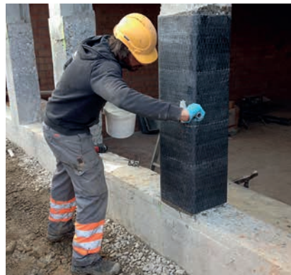
5 Column with S&P C-Sheet 240 (Normal force)
