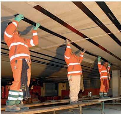
1 Surface applied S&P C-Laminate (Bending)
