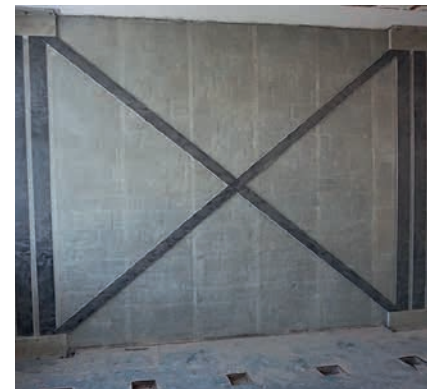
6 Strengthening of masonry with S&P G-Sheet (Seismic enhancement)
