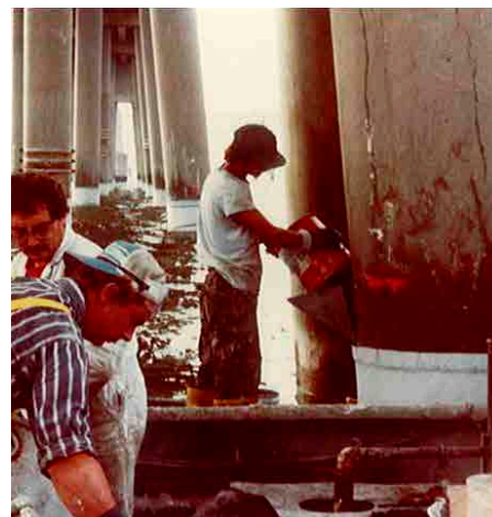
FX-70-6MP™ grout placed in jacket without dewatering
