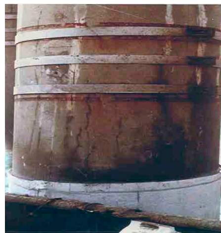
FX-70® System in place and ready for FX-70-6MP™ grout
