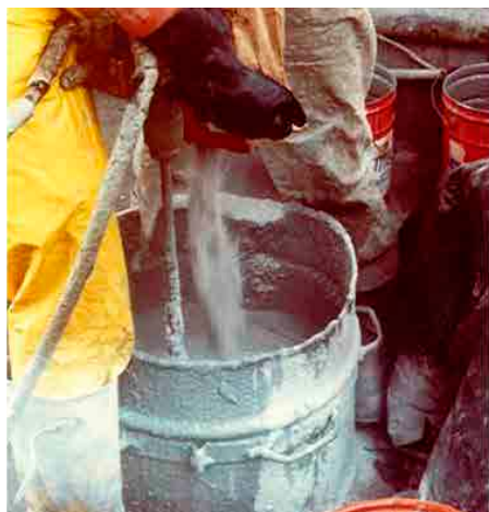
FX-70-6MP™ grout mixed in work boat
