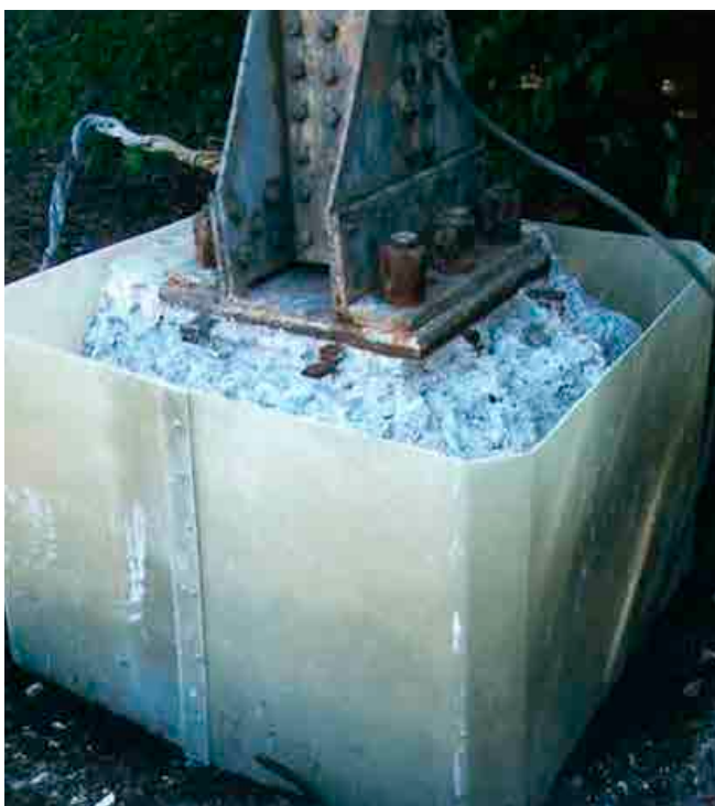
FX-70® jacket installed and backfilled
