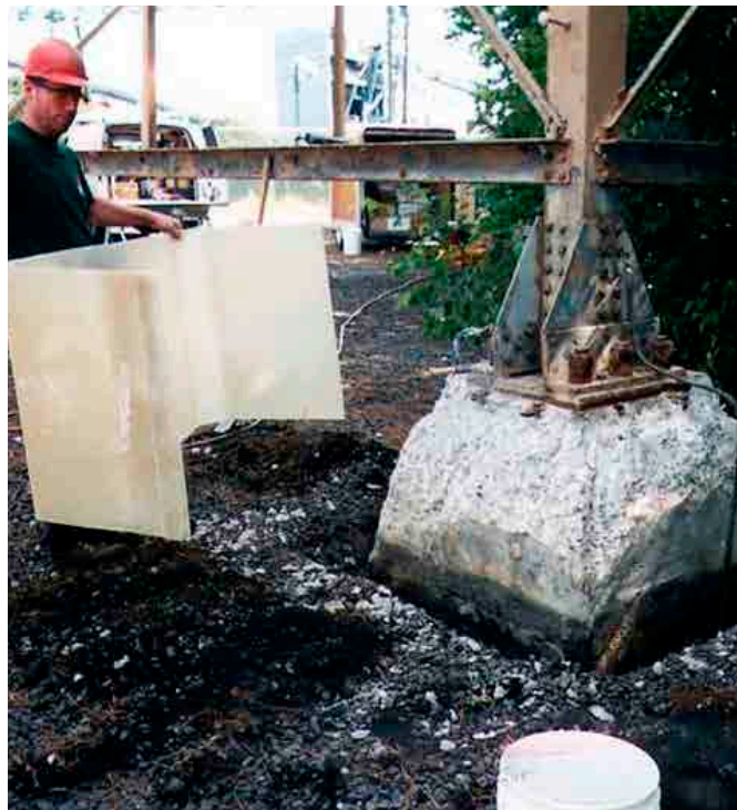
Foundation prepared and excavated; FX-70® jacket installed below ground level for additional protection
