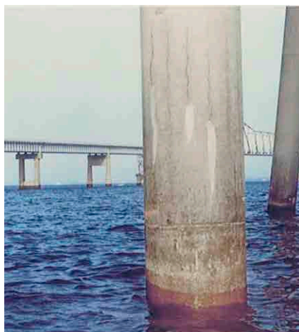
Example of pile "scour"
