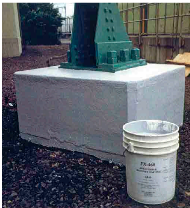
Repair completed with FX-70-6MP™ Multi-Purpose Marine Epoxy Grout as the bottom and top seal material. Coating system is used as a final finish on the outside of the FX-70® jacket.
