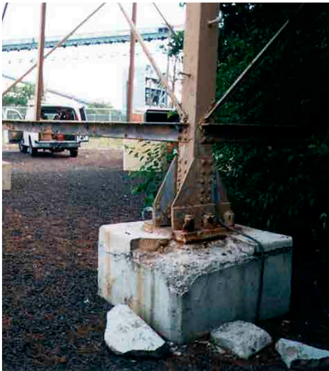
Severe damage to concrete foundation
