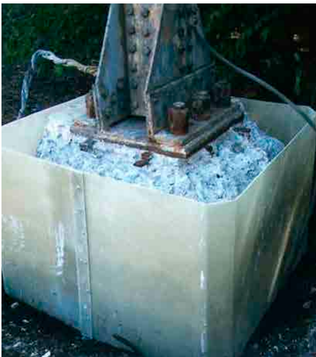
FX-70® jacket installed and backfilled
