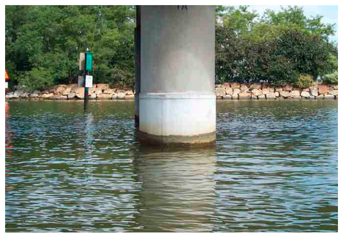
Close-up of a repaired pile; in service 30 years
