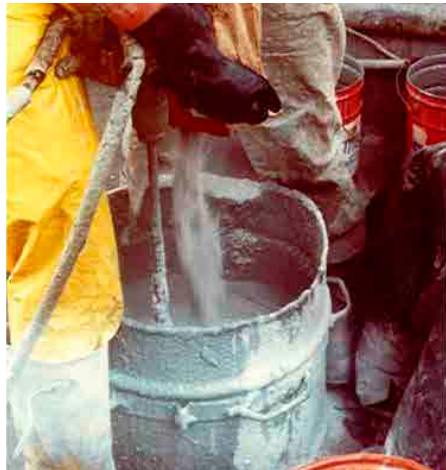
FX-70-6MP™ grout mixed in work boat
