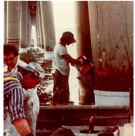
FX-70-6MP™ grout placed in jacket without dewatering
