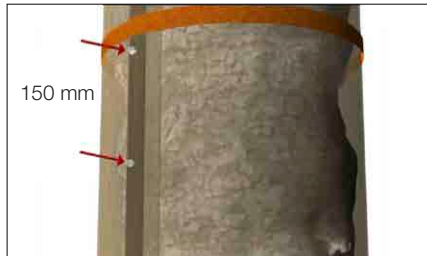
Install a stainless steel, self-tapping screw every 150 mm o.c. to secure the tongue-and-groove joint.
